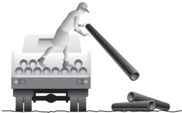
Incorrect way to off-load
