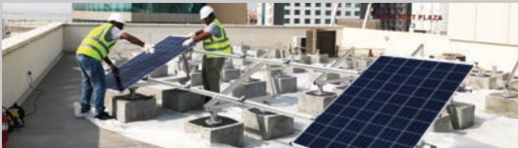
Green Innova installs roof top solar system at MSCEB Headquarter.
