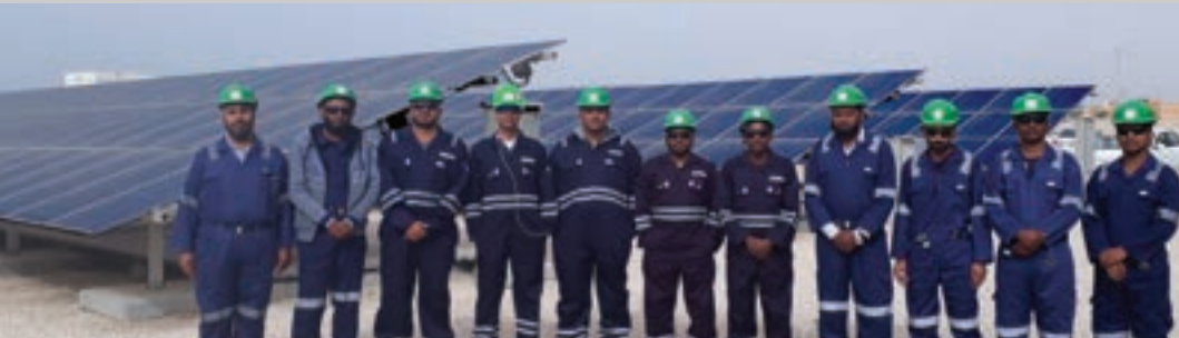
Green Innova conducts O&M activities for solar system at Bapco.
